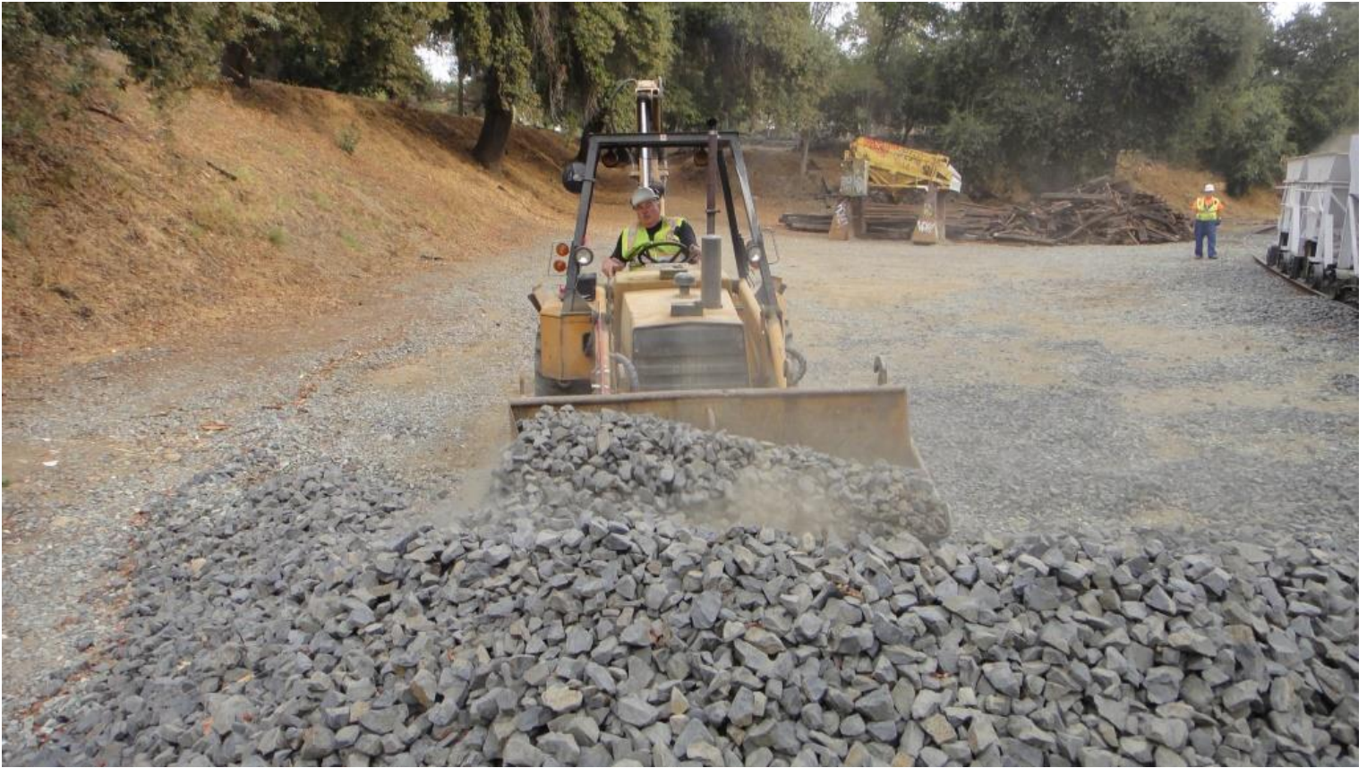
Harry scoops-up a bucket full of ballast rock with the back-hoe...
