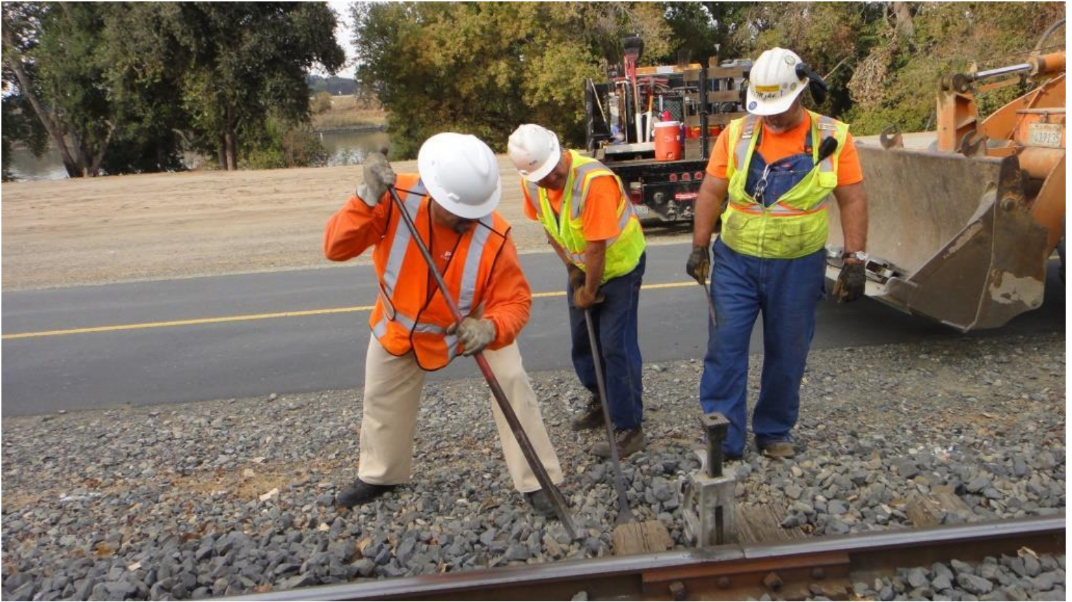
John nips-up a tie while Jose hand-tamps some rock under it to hold it up against the base of the rail
