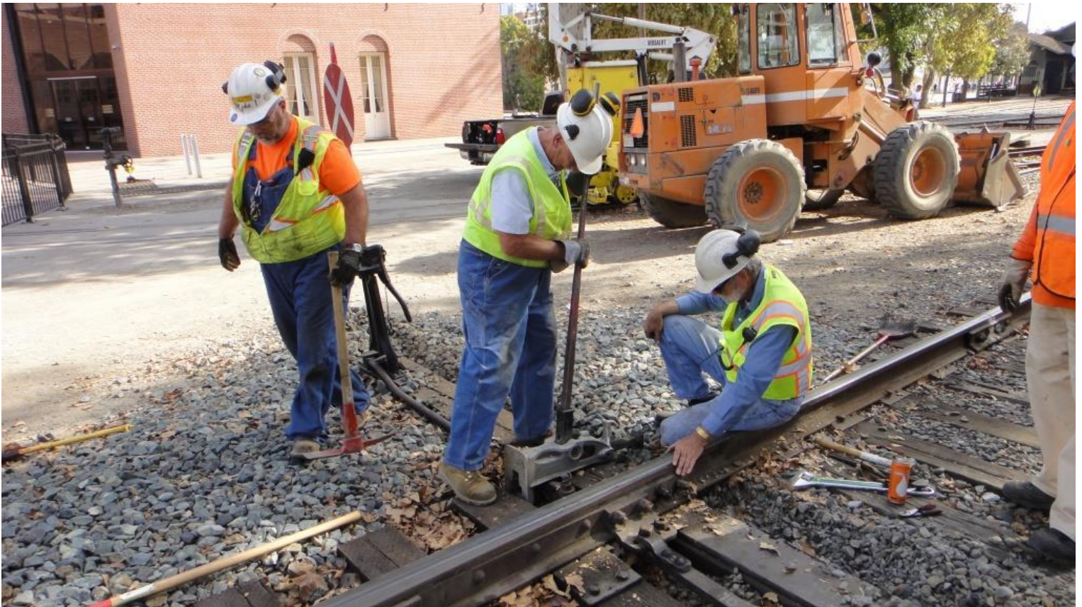
Clem uses a track-jack to push the head-block away from the next tie
