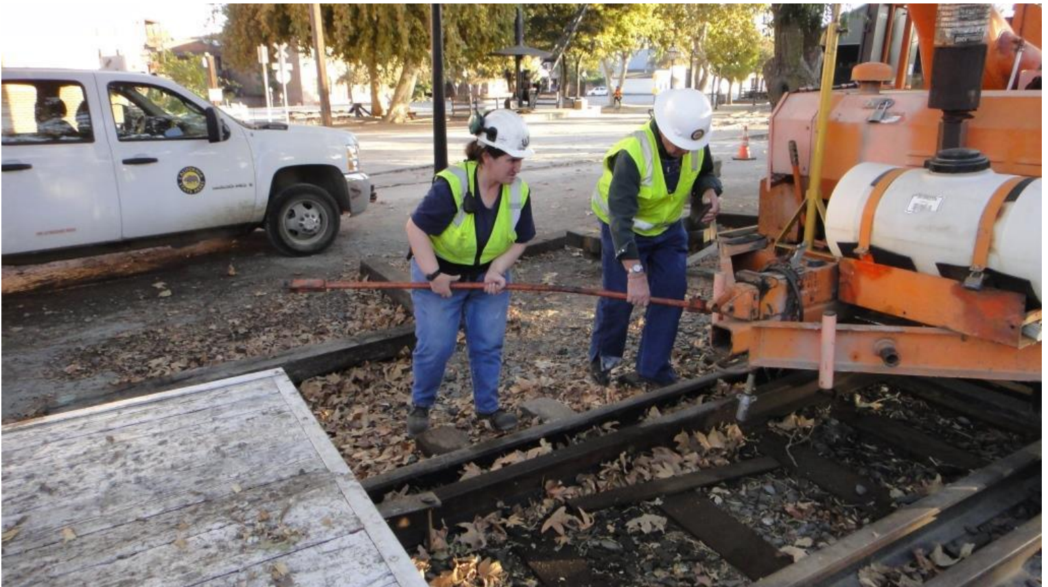
Heather and Cliff put the long draw-bar onto the chipper
