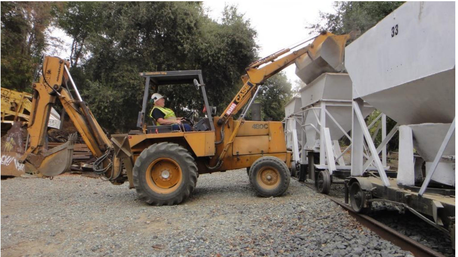
...And deposits it into the a hopper car
