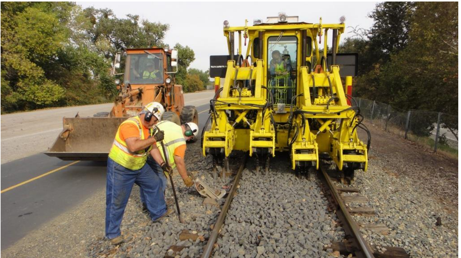
Alan tamps the track to the new level while Frank pulls a jack and Mike F. nips a tie
