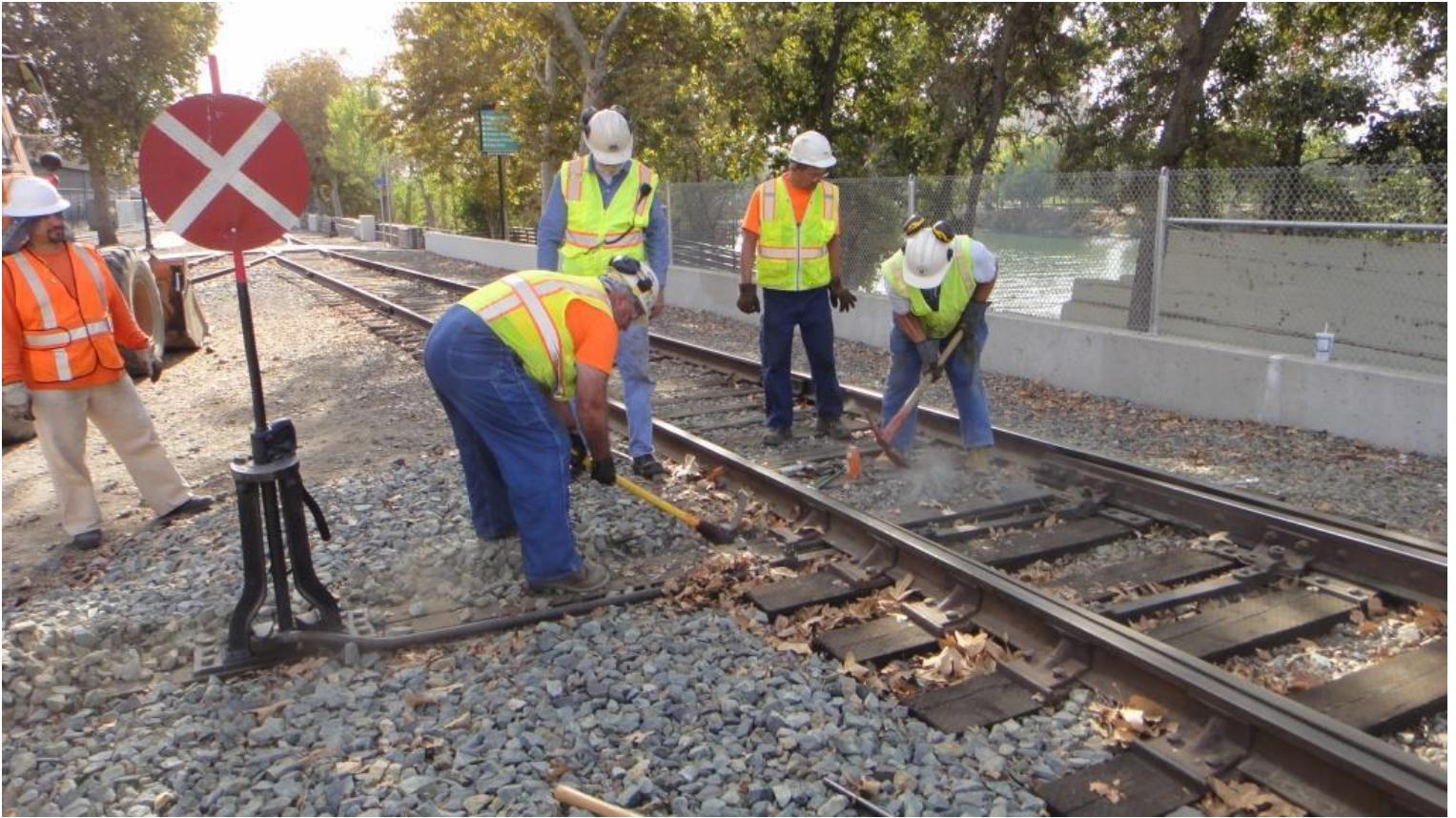
Mike F. and Clem dig-out the south side of the head-block at Switch 101
