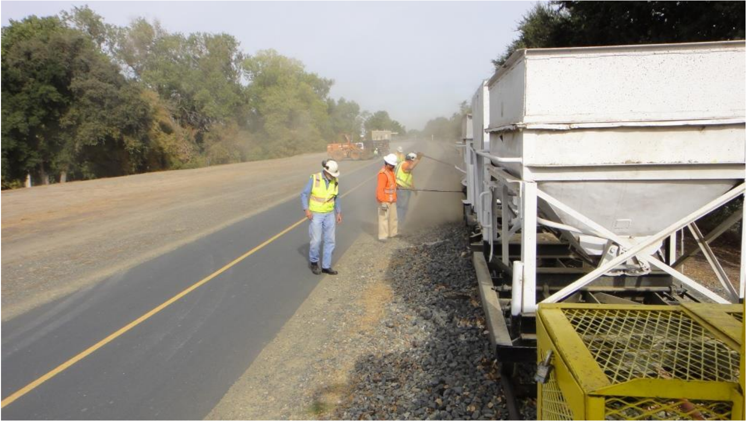
Frank and Jose drop rock from the side-dump hopper
