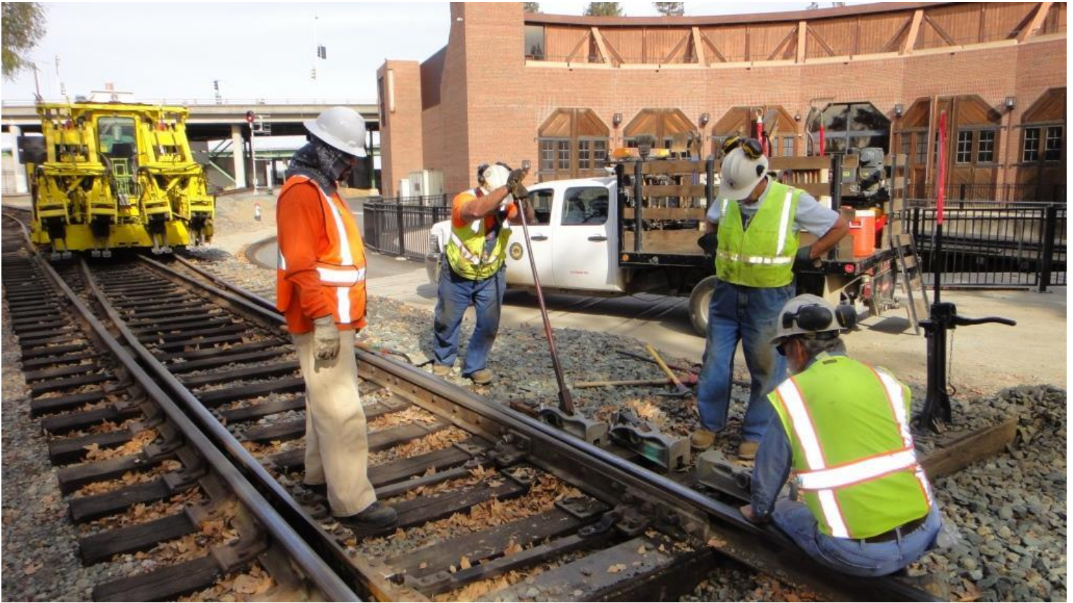
Now, Mike F. move other ties within the switch to position everything properly
