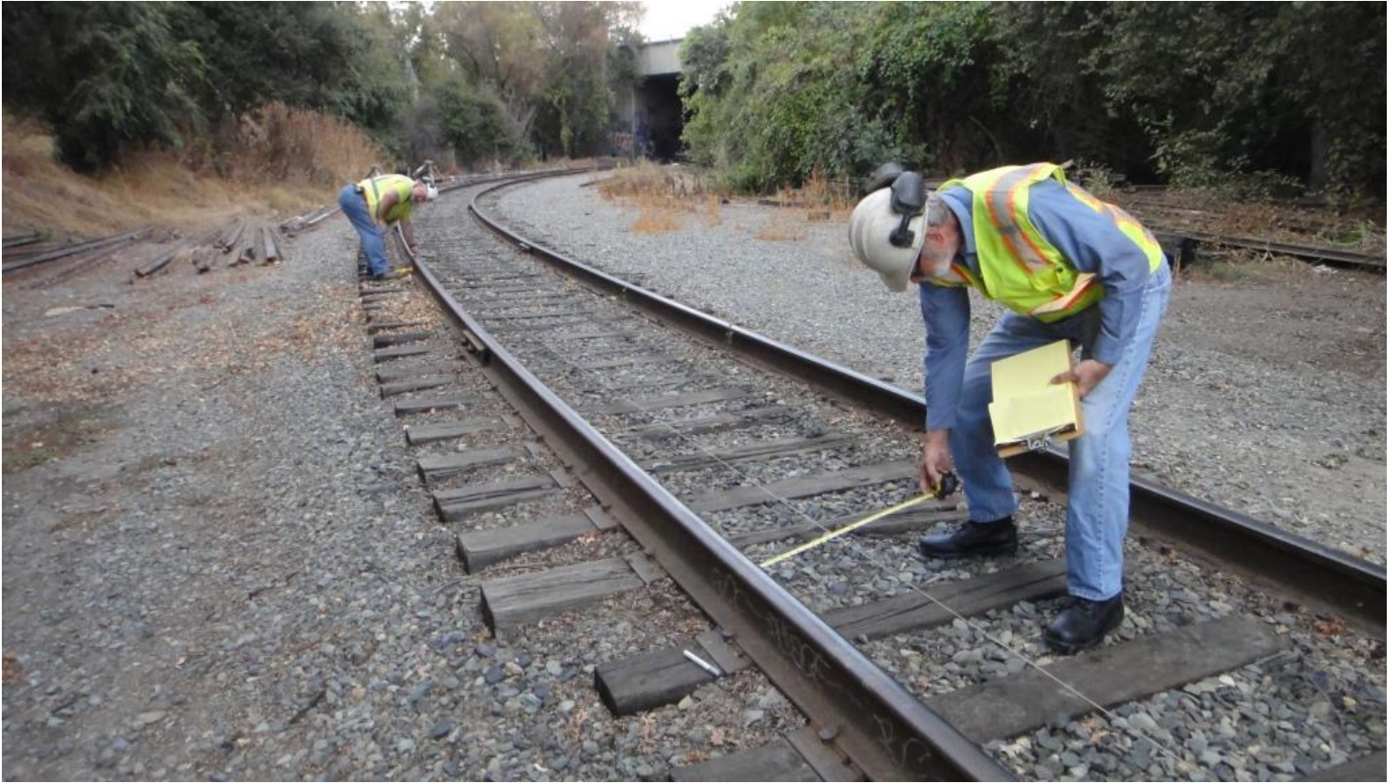
String-lining the curve: Frank hold one end of the string tight as Alan measures the distance between it and the rail at the string's midpoint
