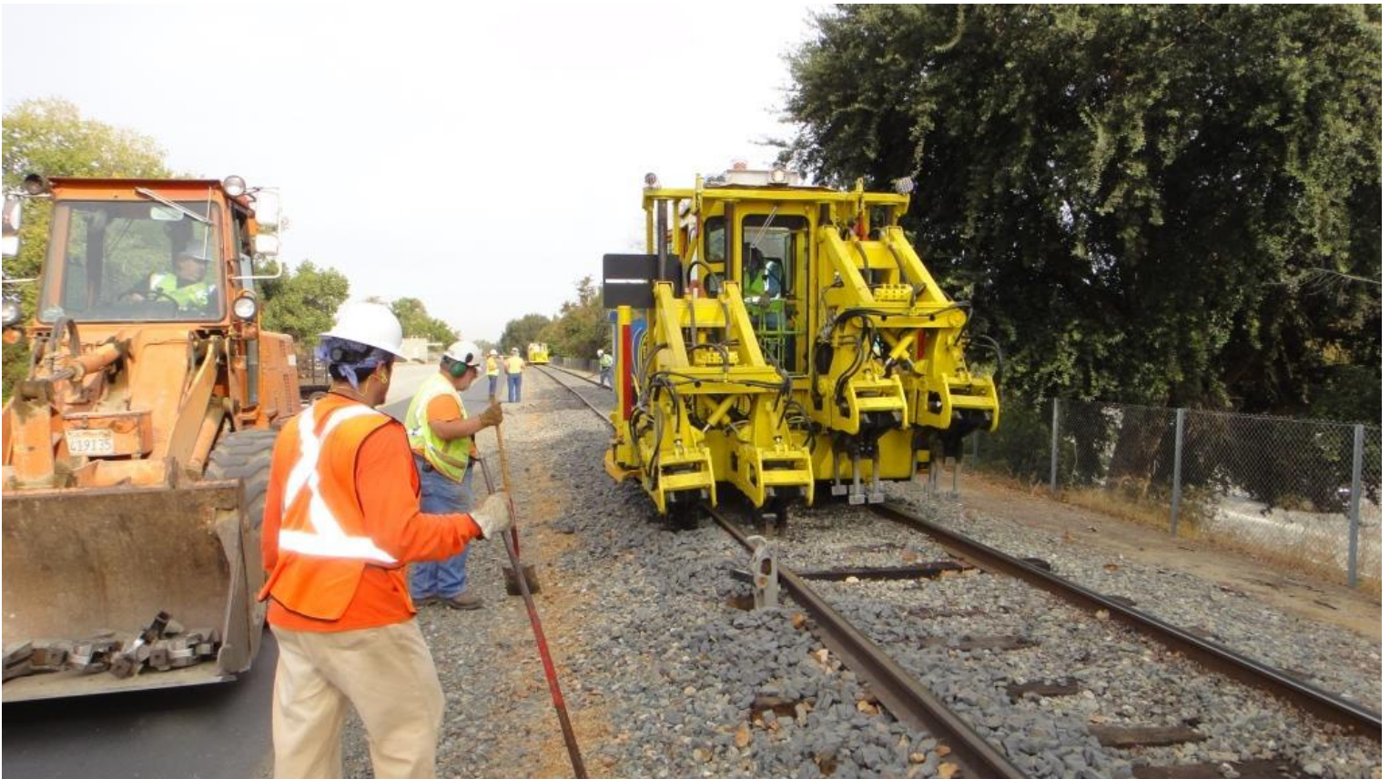
Alan tamps the west rail in a spot where it was exceptionally low
