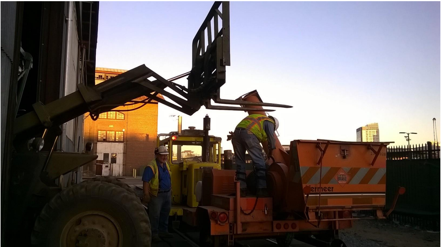
The Green Machine emerges from the south end of the Boiler Shop as Frank and Mike T. get the chain-rig in place
