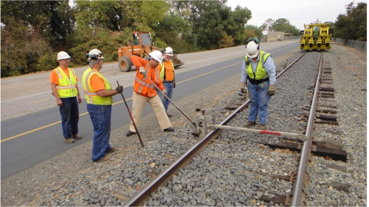
Heather monitors the track-level as Jose jacks-up the west rail
